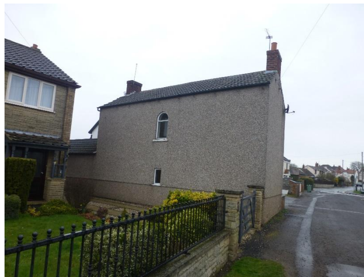
Plate 33: View of 6 Marsh Road looking east
