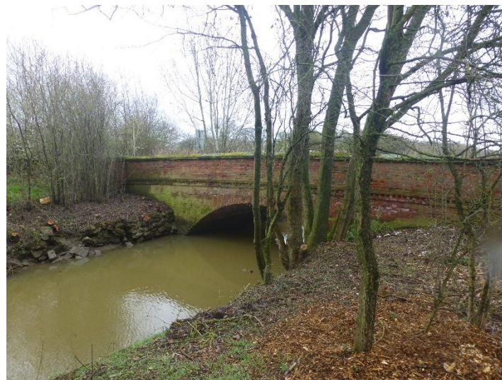
Plate 22: View of bridge adjacent to Dirtness Cottage
