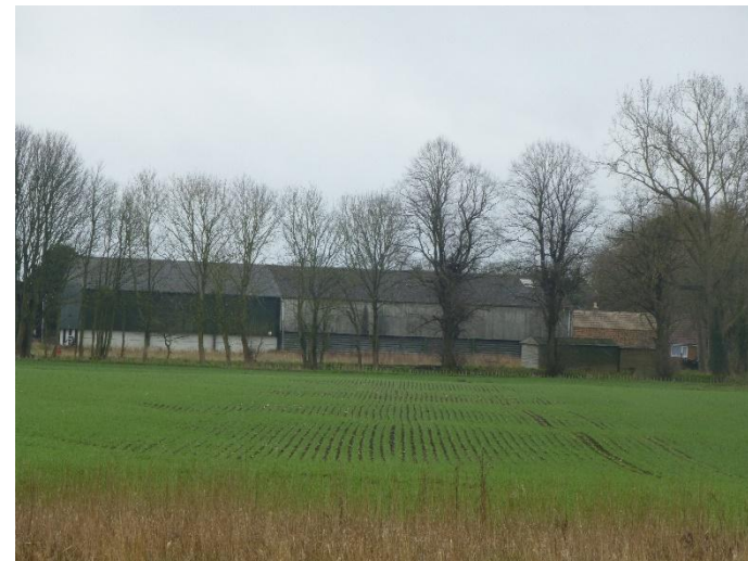
Plate 36: View of Belton Grange looking south
