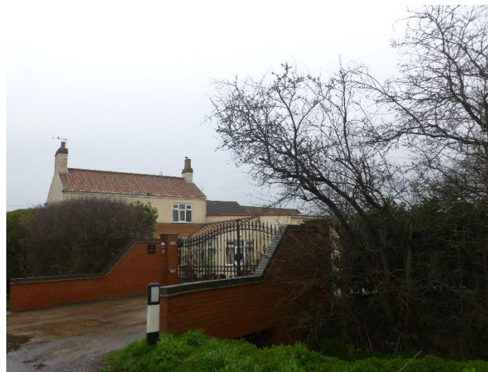
Plate 57: View of The Willows, looking north-east
